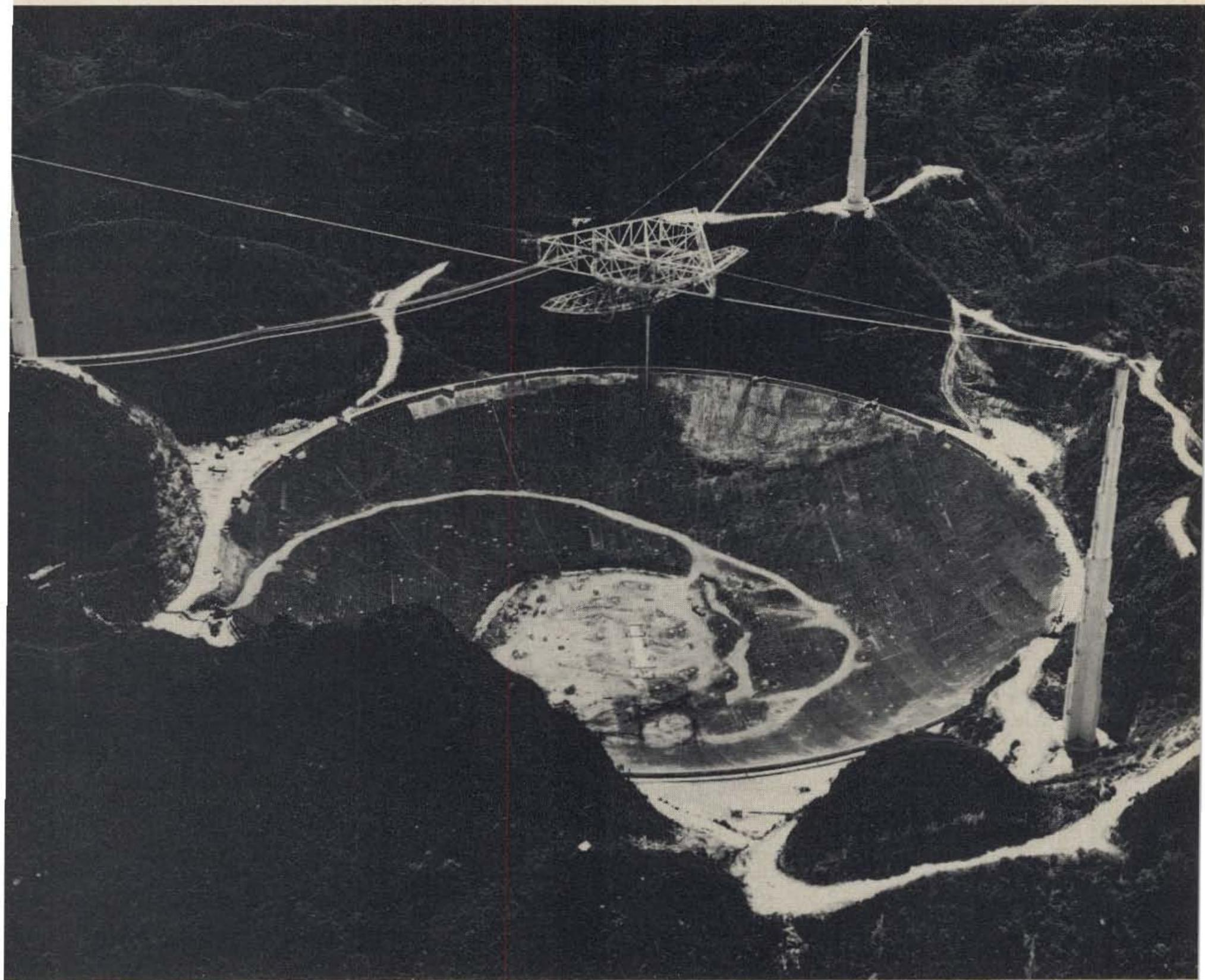
*The giant of all radio telescopes spans some 1000 ft in diameter and 500 ft from the feedhorn to the base. The feedhorn weighs 500 tons and measures 200 ft on each side. Arecibo has been used as both a radio telescope and a radar telescope. The 500-ton feedhorn is supported only by cables. Several contacts via EME with hams in the United States and around the world have been made on the ham bands with the big dish. (Cornell Univ., Arecibo Observatory, Puerto Rico.)*
