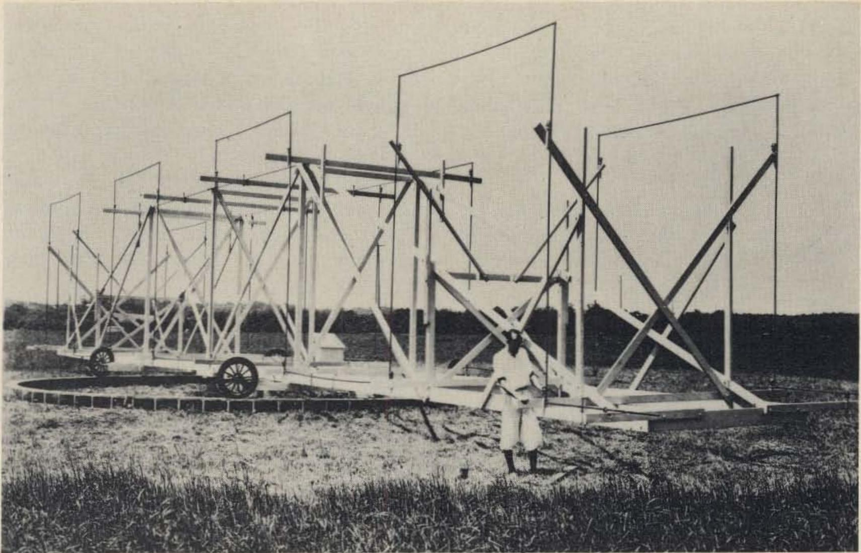
*A historic photo of the late Karl G. Jansky of Bell Telephone Laboratories with the rotating antenna he used to discover radio waves coming from space. Mr. Jansky's investigations during the 1930s into the causes of strange noise in telephone equipment resulted in the discovery of radiation noise from the center of the Milky Way and gave the world a new science — radio astronomy. (Bell Labs.)*
