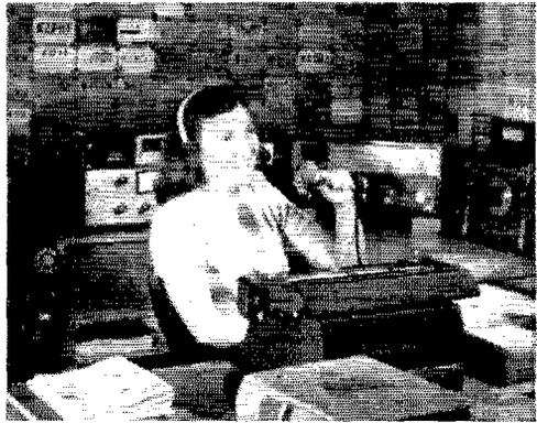
W1ICV's DXCC record is 80 countries worked, 153 confirmed. Jane's OM, W1OOS, is also DXCC with 200 countries plus. The DXing Andersons of Terryville, Conn., use an HT-30 exciter, HT-31 linear and another linear amplifier using a pair of 4-400As. They receive with an HRO-60 and have beams on 20 and 10 and doublets on 80 and 40.
