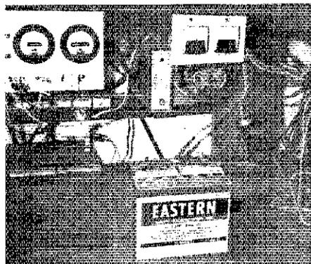
The meter panel and batteries located in the radio room are convenient to the repeater power supply. To the right is the repeater power panel. On the floor is a 60-Ah (ampere-hour) battery that powers the repeater. To the left is the windmill panel which monitors generator voltage, load current and regulator condition. (Photo courtesy MWO)
