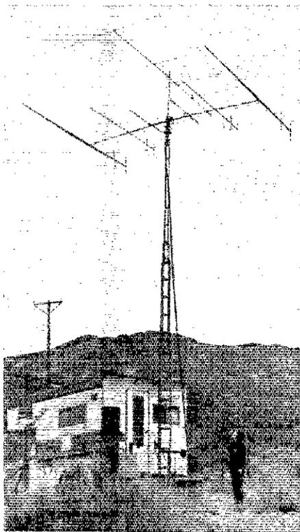
In this photo WB6IDK looks over an array of two quagis each for 144, 222 and 432 MHz (plus a five-element Yagi for 50 MHz) at a site in southwestern Utah. From this site K6YNB/7 worked numerous stations in the Los Angeles area, 400 miles away, on all bands through 432. A *nonconductive* support is recommended when quagis are mounted side-by-side as here.
