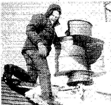
The mill on the roof comprises a Savonius rotor made from trash cans attached to the rear axle salvaged from a truck. Here, Observatory Director Guy Gosselin has stopped the rotor so that he can scrape the rime ice from it. (Photo courtesy MWO)
