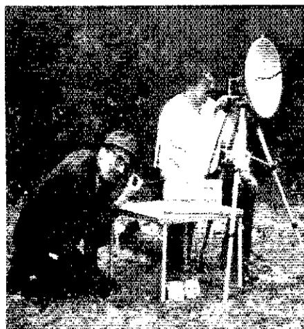
Fig 2—Shown in this picture is the Mt Ashland, Oregon, side of the 47-GHz contact. Roger McCoy, W7ADV (left), listens intently for the WA3RMX/7 signal while John White, K7RUN, aims the 18-inch dish. Roger and John are associated with the Tektronix Employees' Amateur Radio Club. Not pictured, but also involved in setting the new record, is Rick Bremmeyer, WA7GFP.
